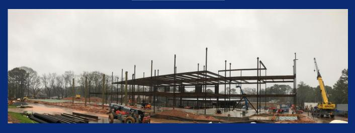
Photo of the project site with sequence 2 & 3 steel in progress
